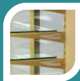
Detail uchycení polic / Detail of shelves holder
