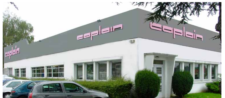
1992 - Usine de Gretz-Armainvilliers 1992 - Gretz-Armainvilliers factory
